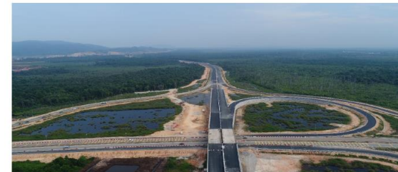
Extension of MCKIP Main Access Road to Northern Link Road 扩展北环路和主要干道
